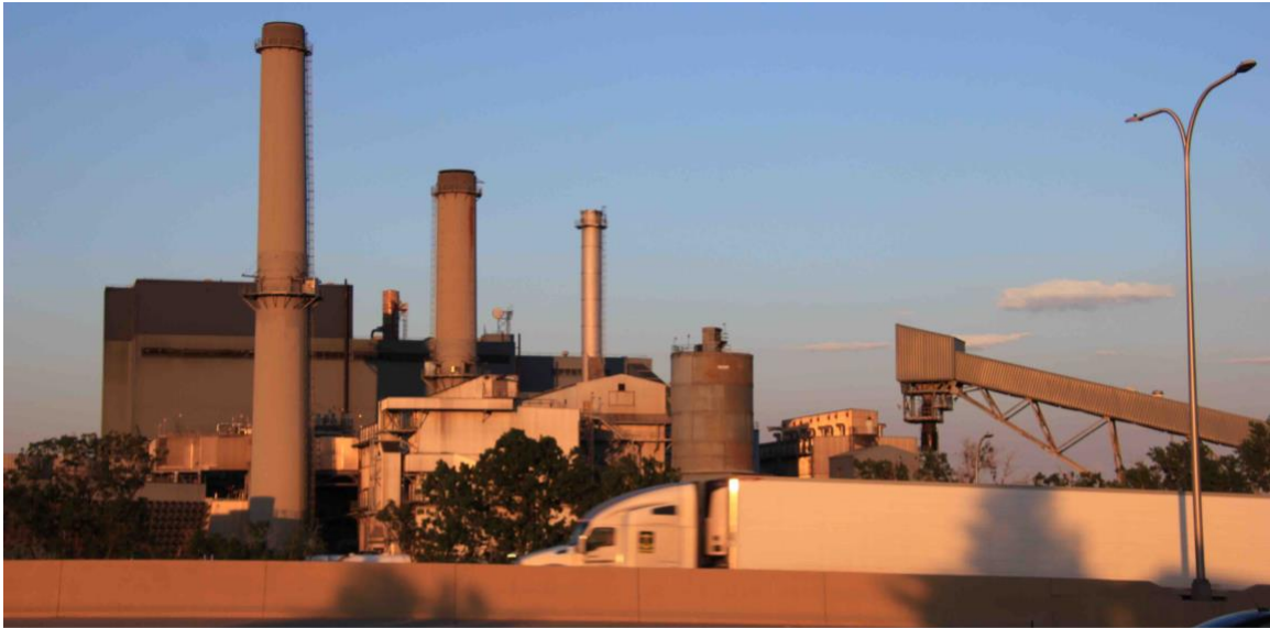
The Martin Drake plant near downtown Colorado Springs is to be closed by 2023 and 7 gas-fired generators moved in to generate power until 2030. Photo/Allen Best
