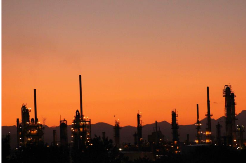
The Suncor refinery in Denver. Photo/Allen Best
