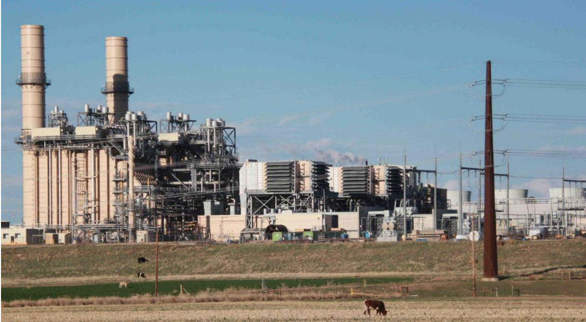
A gas-fired power plant northeast of Denver. Photo/Allen Best
