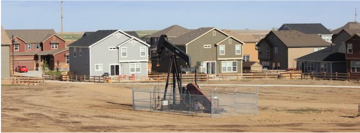
A pumping jack surrounded by housing at Dacona, Colo.
