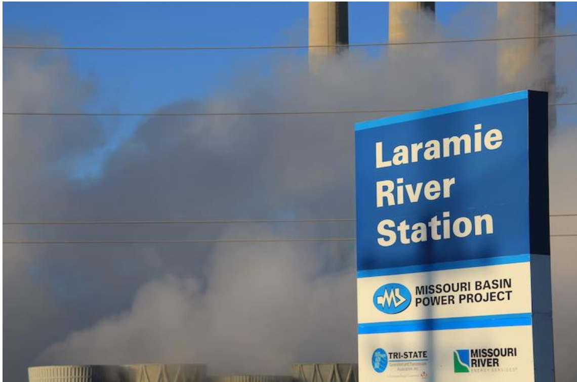
Tri-State Generation and Transmission has upped its stake in the Laramie River Station near Wheatland, Wyo., motivated primarily because of the added transmission the deal gives it, according to a filing. Photo/Allen Best
