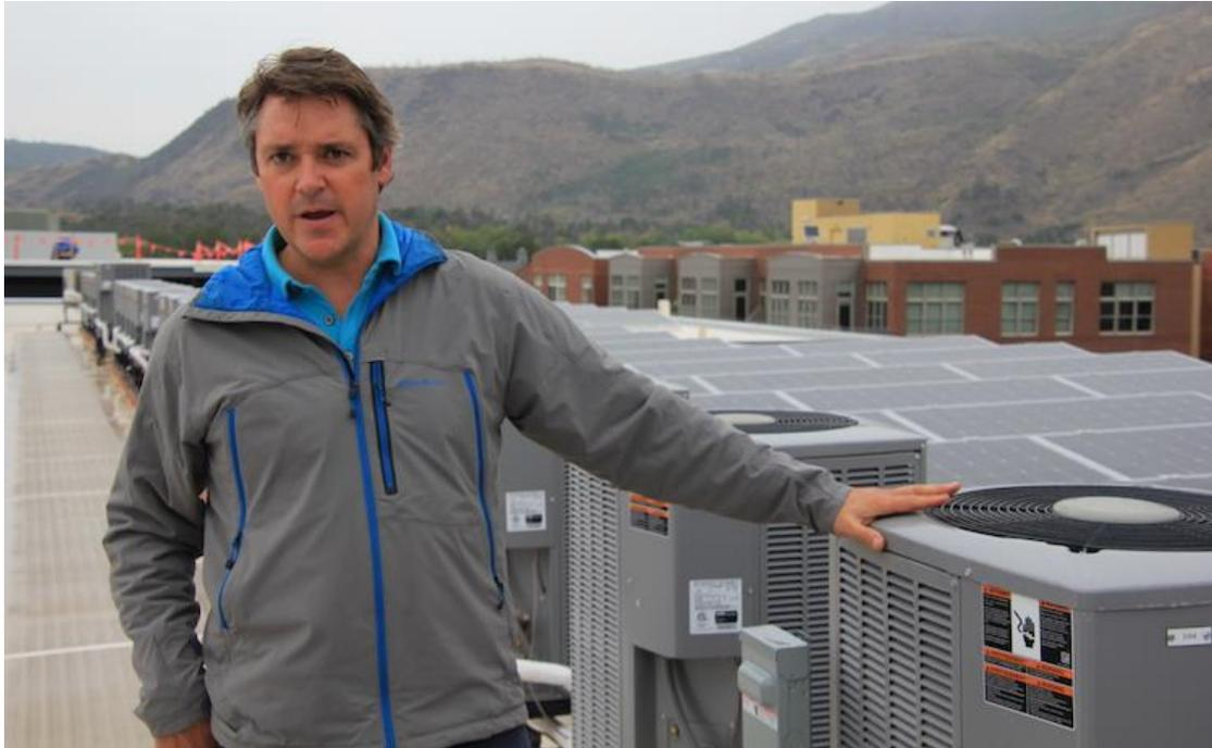
**Philip Jeffreys, project development manager for The Hub, the Aspen Skiing Co.'s all-electric employee housing building at Basalt, explains the array of roof-top air-source heat pumps and solar panels that allow the building to perform without need of natural gas.**
