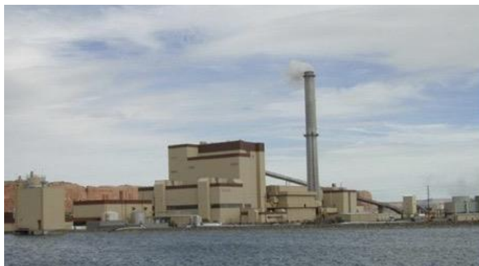
The Springerville coal plant. Photo/Tri-State G&T
