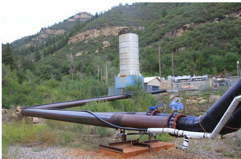
Electricity was produced for several years at the Elk Creek Mine near Paonia, but too little methane remains to be effective.
